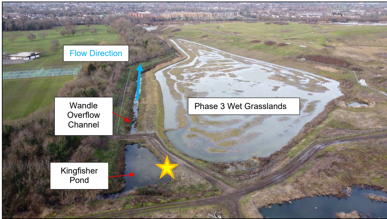
Figure 4 Phase 3 Wet Grasslands Viewed looking West
